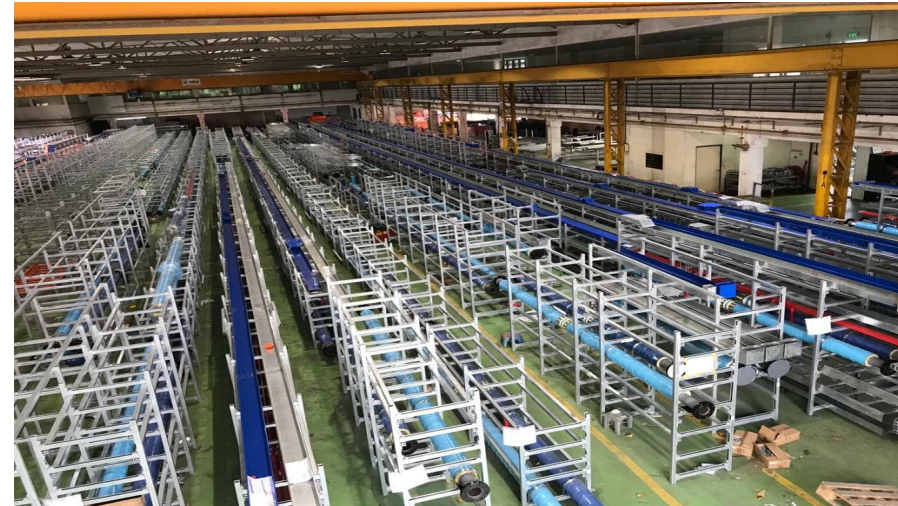
Modular M&E services installation
